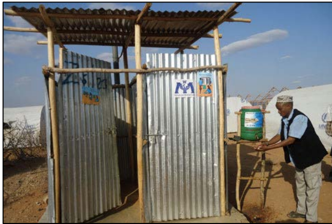
Figure B30: Latrine Construction in a refugee camp (IMC, No Date)
