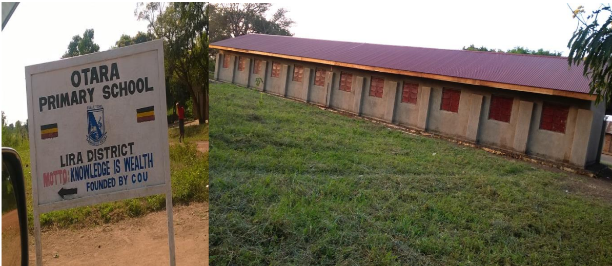
Classroom constructed at Otara P/S under phase I schools
