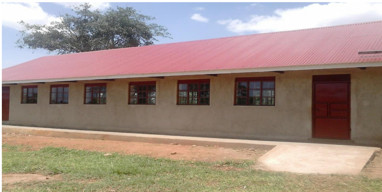
Classroom constructed at Bishop Hanington P/S in Mayuge District under phase I schools
