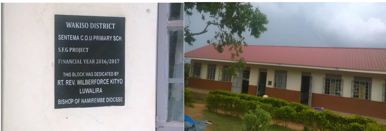
Classroom constructed at Sentema C.O.U in Wakiso District under phase I schools
