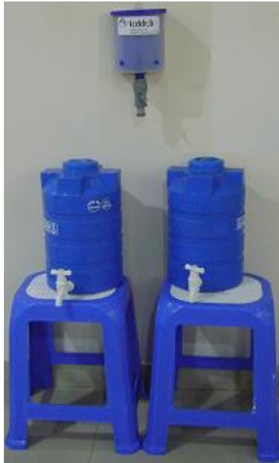
Figure 1: The chlorine dispenser hardware
