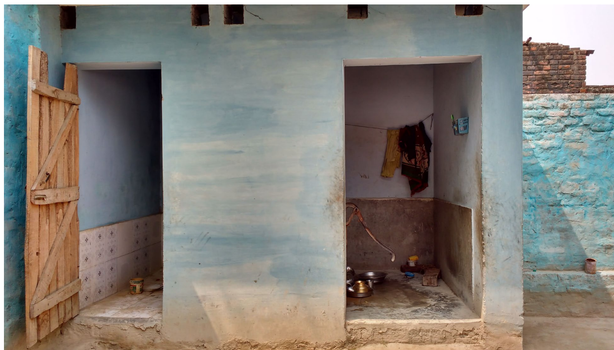
Figure 5: Toilet constructed per SBM guidelines, no reimbursement received, Paschim Champaram
